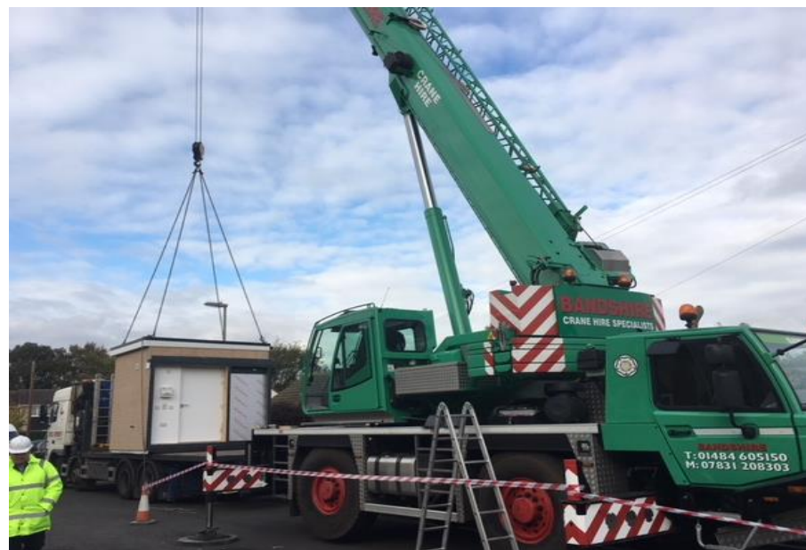
The POD Being Craned In
